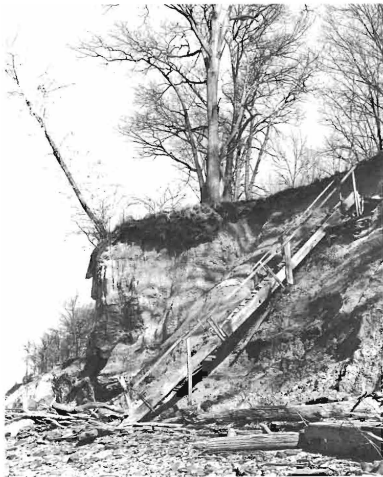
Coastline near Grove Point in Upper Chesapeake Bay.
