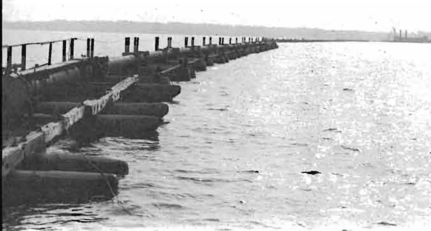
Open-water pipeline dredging operation in Upper Chesapeake Bay.
