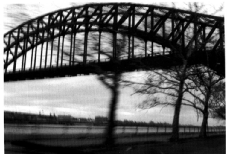
Railroad Bridge from Queens, NY, 1998 Black and white photograph, 8 x 10"
