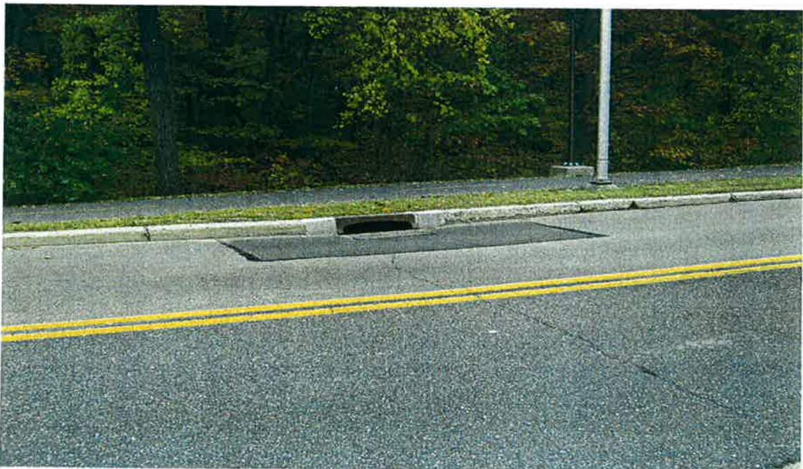
Photograph No. 10: View of a curbside storm drain along Circle Road, looking east. The subject property is located at the upper half of the photograph.
