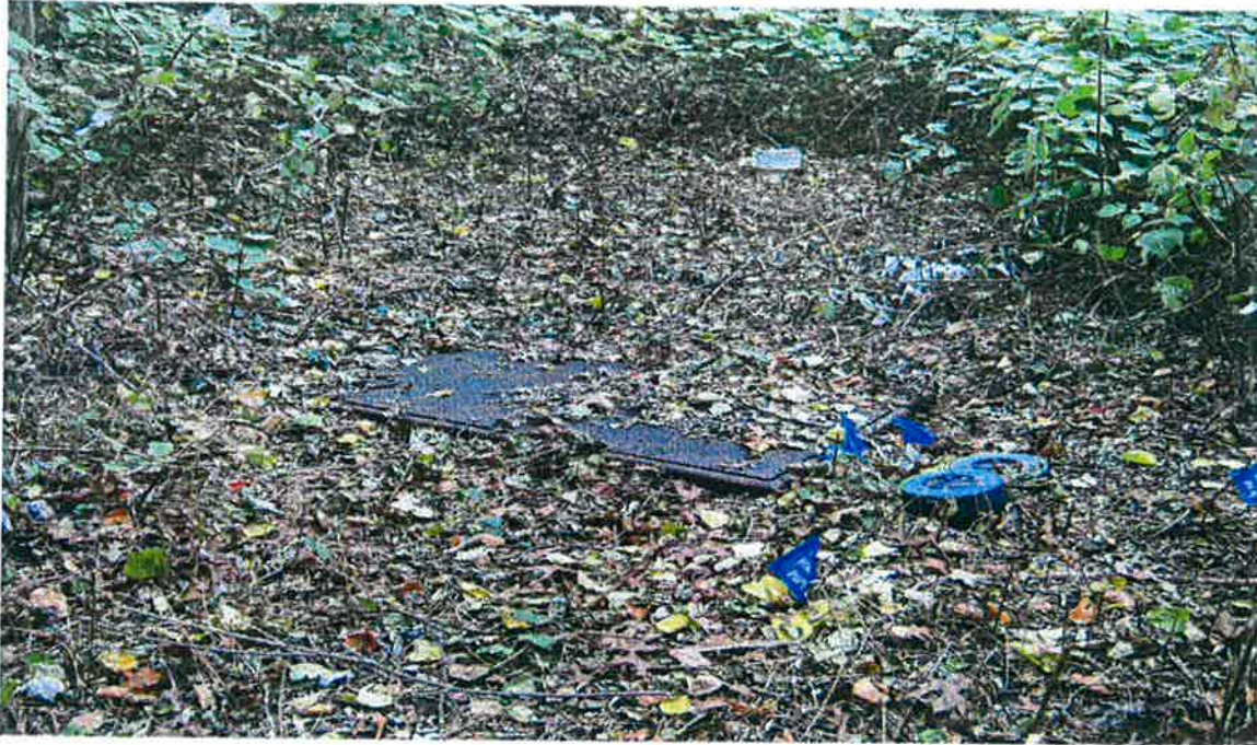
Photograph No. 9: View of a sub-grade utility vault near the southern boundary of the property.
