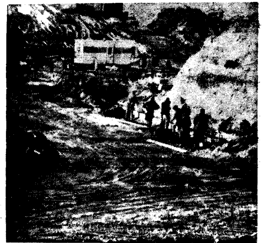
Workers at the Campus Center construction site before the blizzard.
