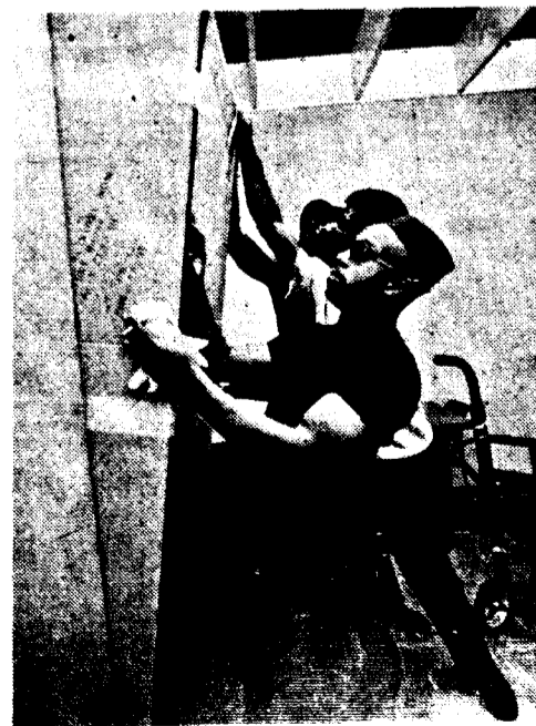
INMATES FROM THE BEDFORD HILLS DETENTION CENTER are installing shelves in the Library.
