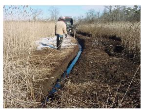
Figure 5 - Pisten Bully creating tidal channel along landward side of Area 1. In order to mitigate potential spreading of *Phragmites*, the soil from tidal channel along this portion of the marsh was deposited upland into an existing *Phragmities* stand. Environmental monitor in foreground.
