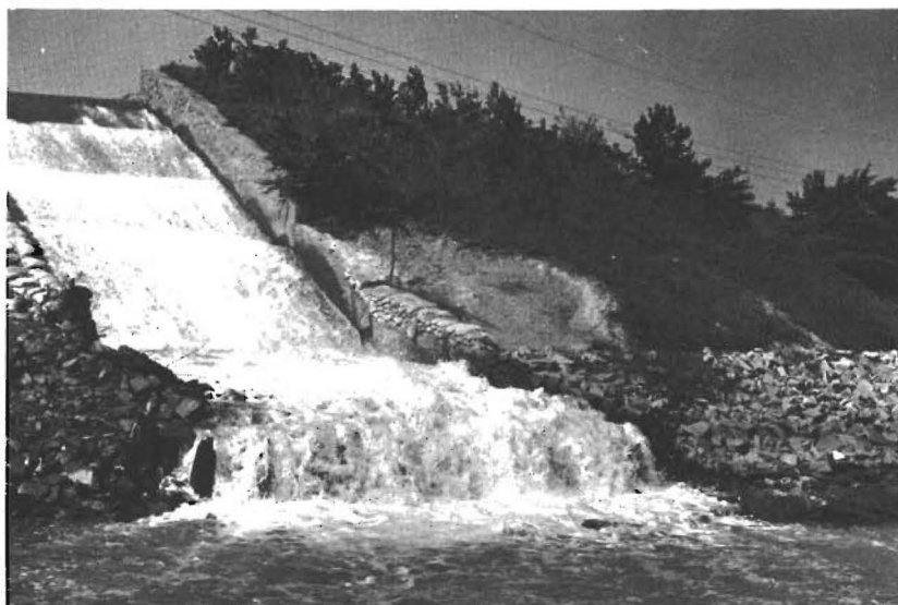
Fig. 22. Spillway, showing discharge entering north side of the Canal.
