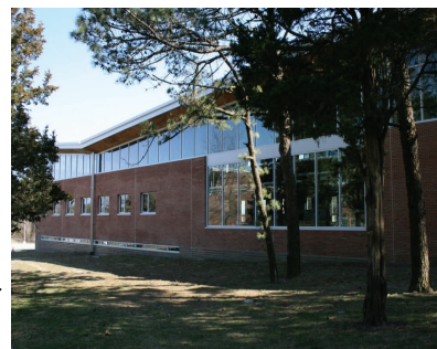
South Face of New Building
