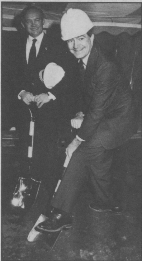
DIGGING IN. President Marburger, with the help of Congressman George Hochbrueckner, turns shovels full of soil east of Nicolls Road. Over the next few months others will help until a new Veterans Home is completed.
