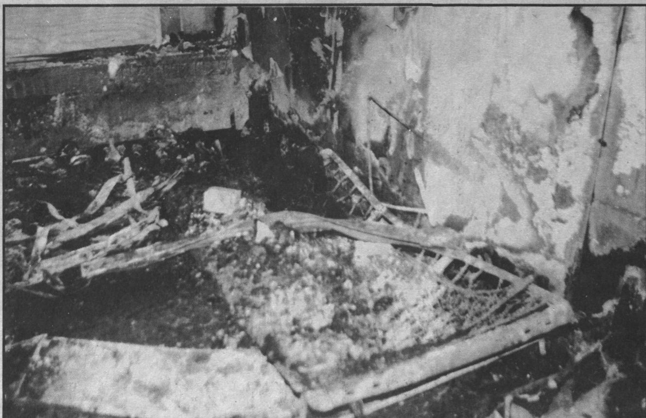
The view from the doorway of the A room in Suite 212. Experts who examined the room said the blaze originated near the small white box near the center of the photo.
