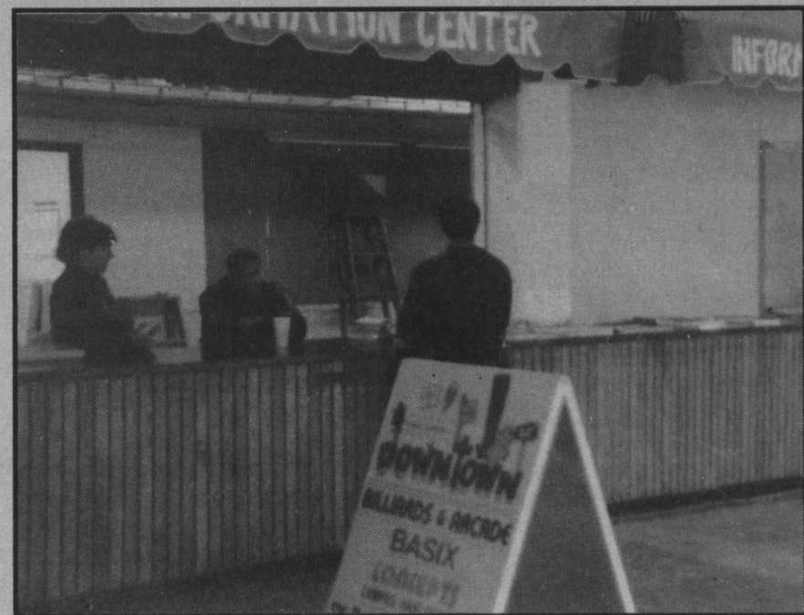
Construction at right of Information Center will be a Public Safety satellite station in the Student Union. According to spokesman Doug Little, the station will make Public Safety more accessible to students.
