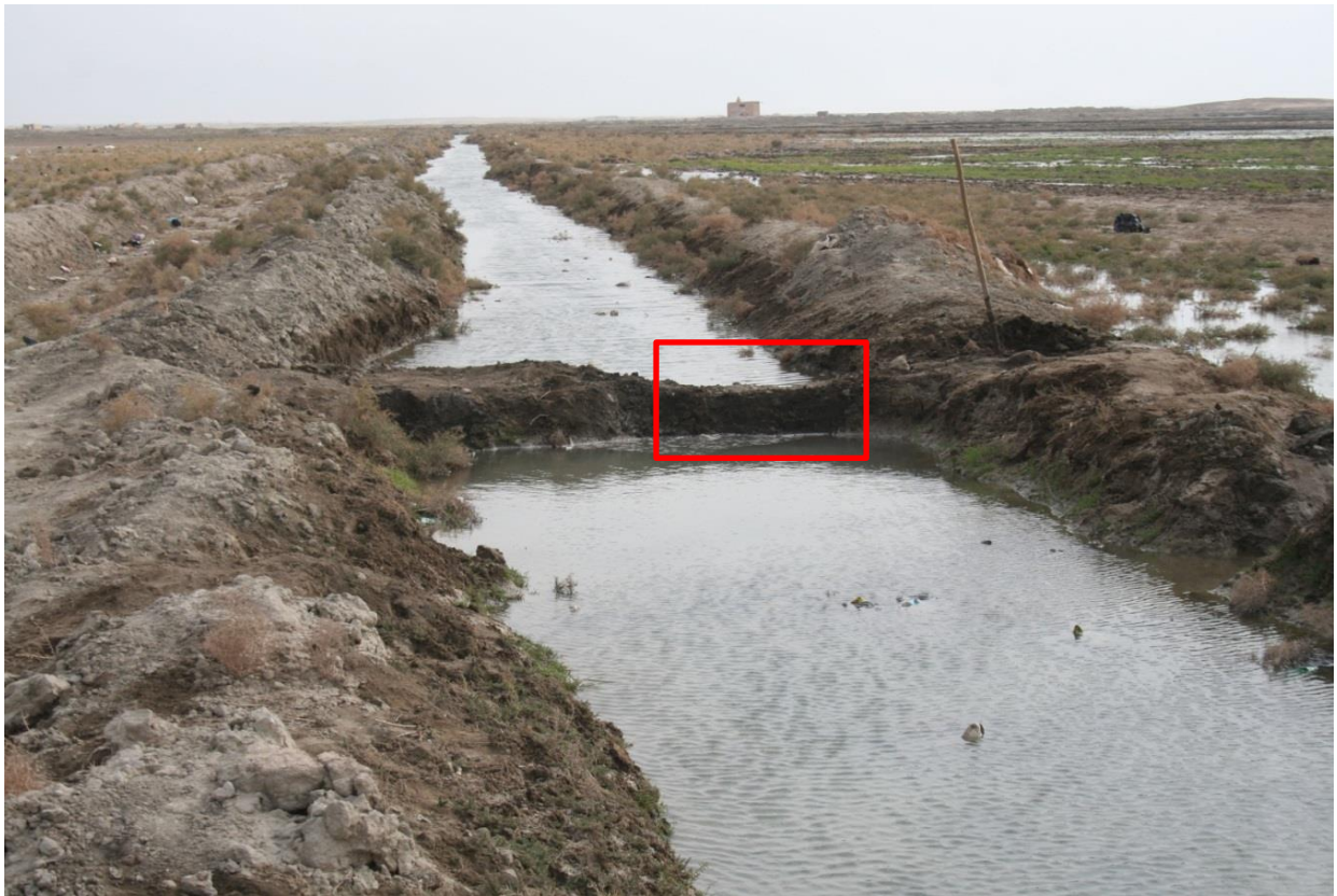
Figure 2.8 Control dam to regulate the water flow within a canal
