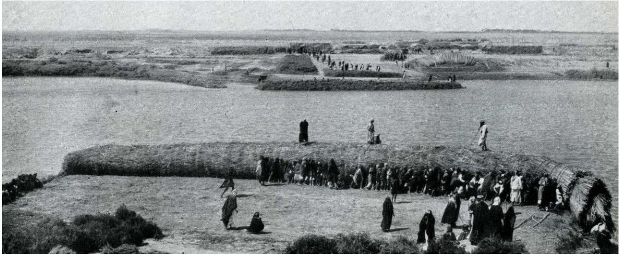
Figure 2.6 a Reed dam to block the Euphrates River, 1909 (Great Britain Admiralty 1944: 436)
