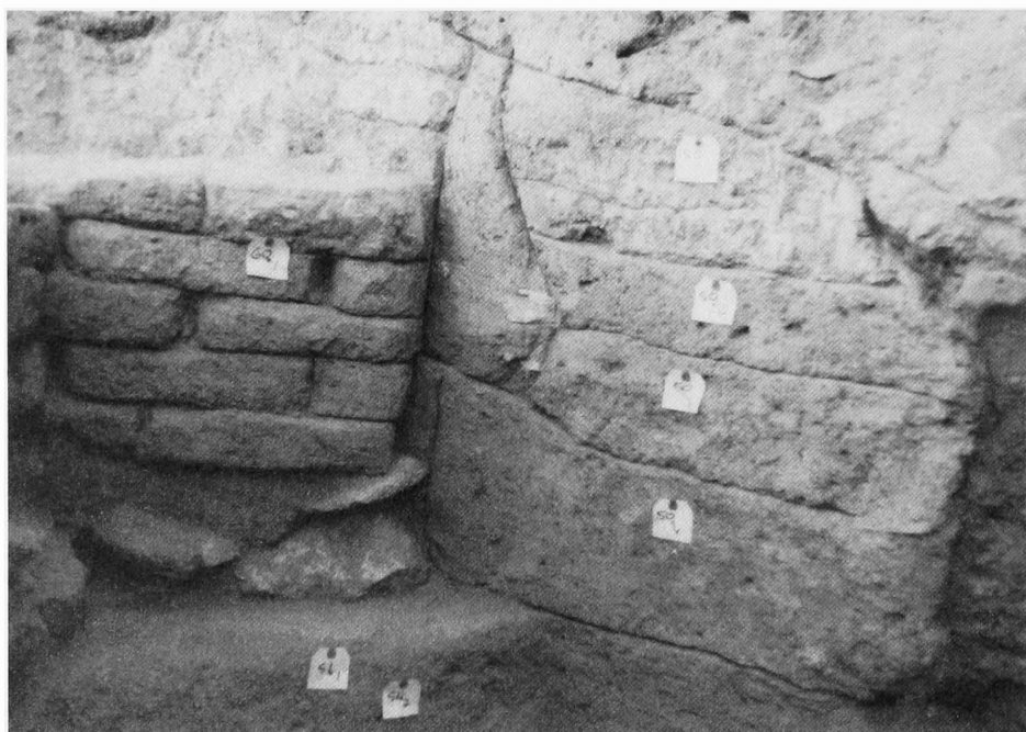
Fig. 2.5. Doorway in the northwestern wall of the NE Building in Operations 1, 20 and 12, Phase 2, with the floors and plasterings associated with the original and secondary rebuilding of the NE Building detailed.
