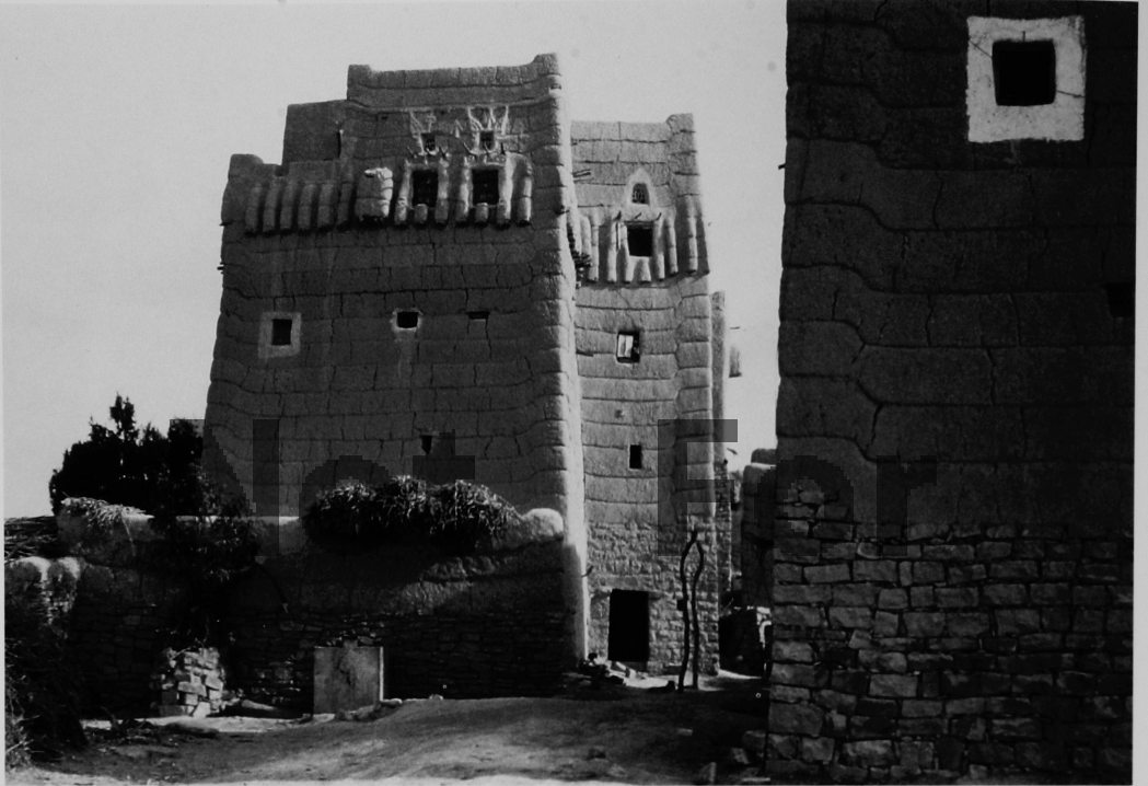
a. Typical Exposed Zabor Construction.
