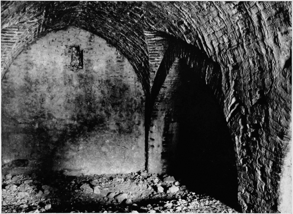
(b) Detail of vaulting in hân.
