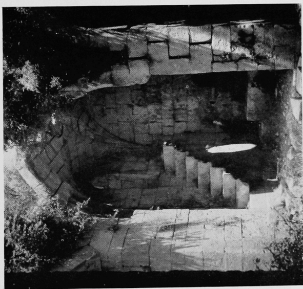
(a) Staircase in Alara Hân, p. 46.
