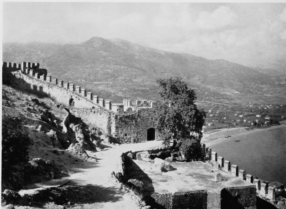
(b) Kale Kapısı seen from the interior. In the foreground the sarnıç.
