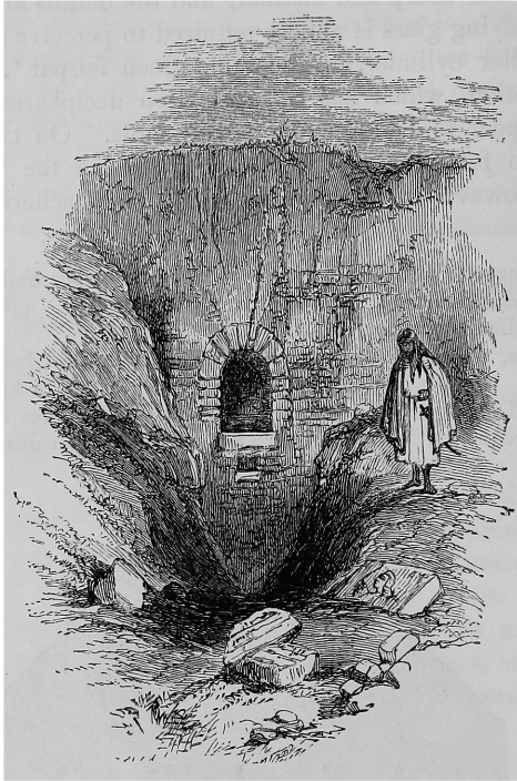
Vaulted Drain beneath the North-west Palace at Nimroud
