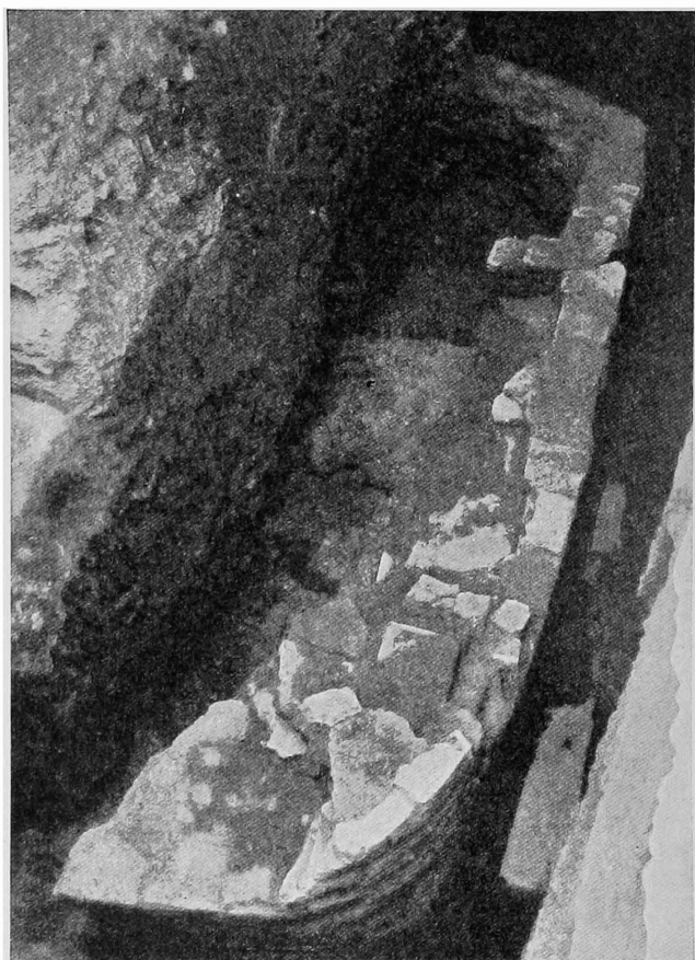
FIG. 122.—The western pier of the bridge over the Euphrates.
