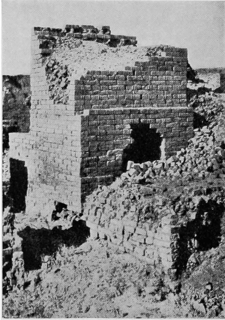
FIG. 71.—Wall of two-ridged bricks in Southern Citadel.
