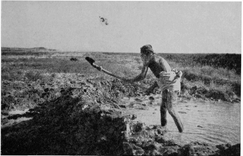
FIG. 10.—Arab at work on a canal, in the neighbourhood of Babylon.
