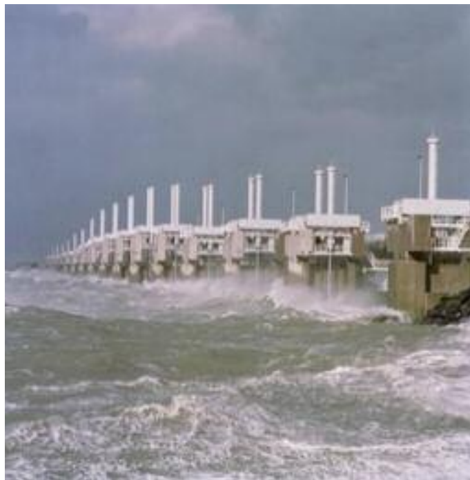
The storm surge barrier across the Oosterschelde estuary at work during a storm.
