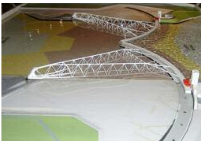
Scale model of the Maeslant Barrier. The ocean is to the right and the port of Rotterdam is to the left of the image. The gates are shown in the storm (closed) position. During fair weather, the gates retract into “parking areas”.
